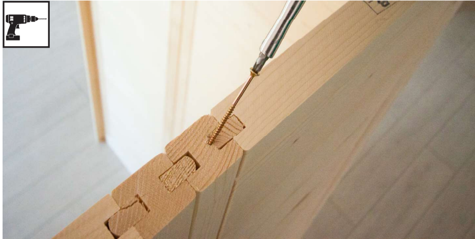
3 mm drill bit, 4 screws 4 x 70 mm
